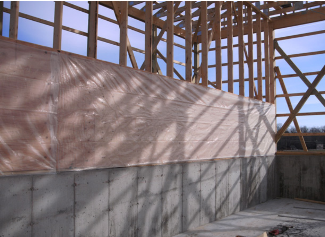
Figure 19: Vapor Barrier on Back Push Wall at UNH Composting Facility
