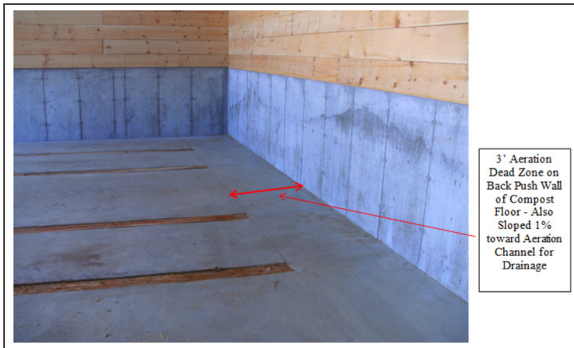
Figure 8: Aeration Floor Spacing for UNH Compost Facility
