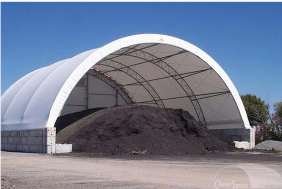
Figure 20: Example Compost Setup Utilizing a High-Tension Fabric Structure with Waste Block Walls (ClearSpan 2013)
