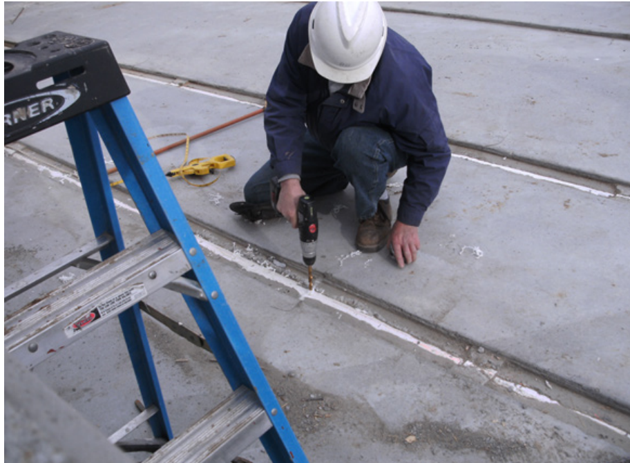
Figure 33: Drilling of Aeration Holes
