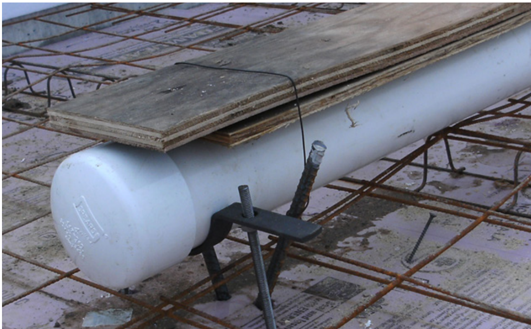
Figure 27: Aeration Line Forms for Cover Plates
