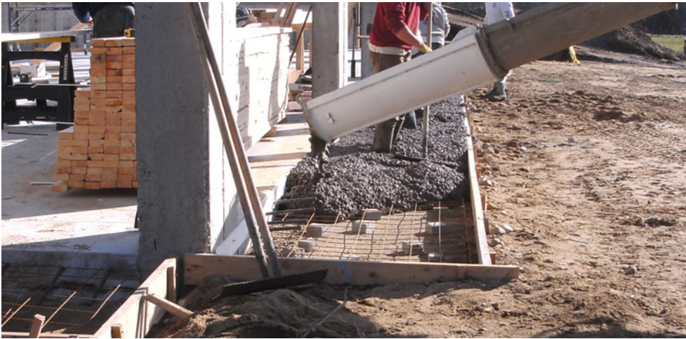
Figure 40: Specifications When Pouring the External Concrete Pad
