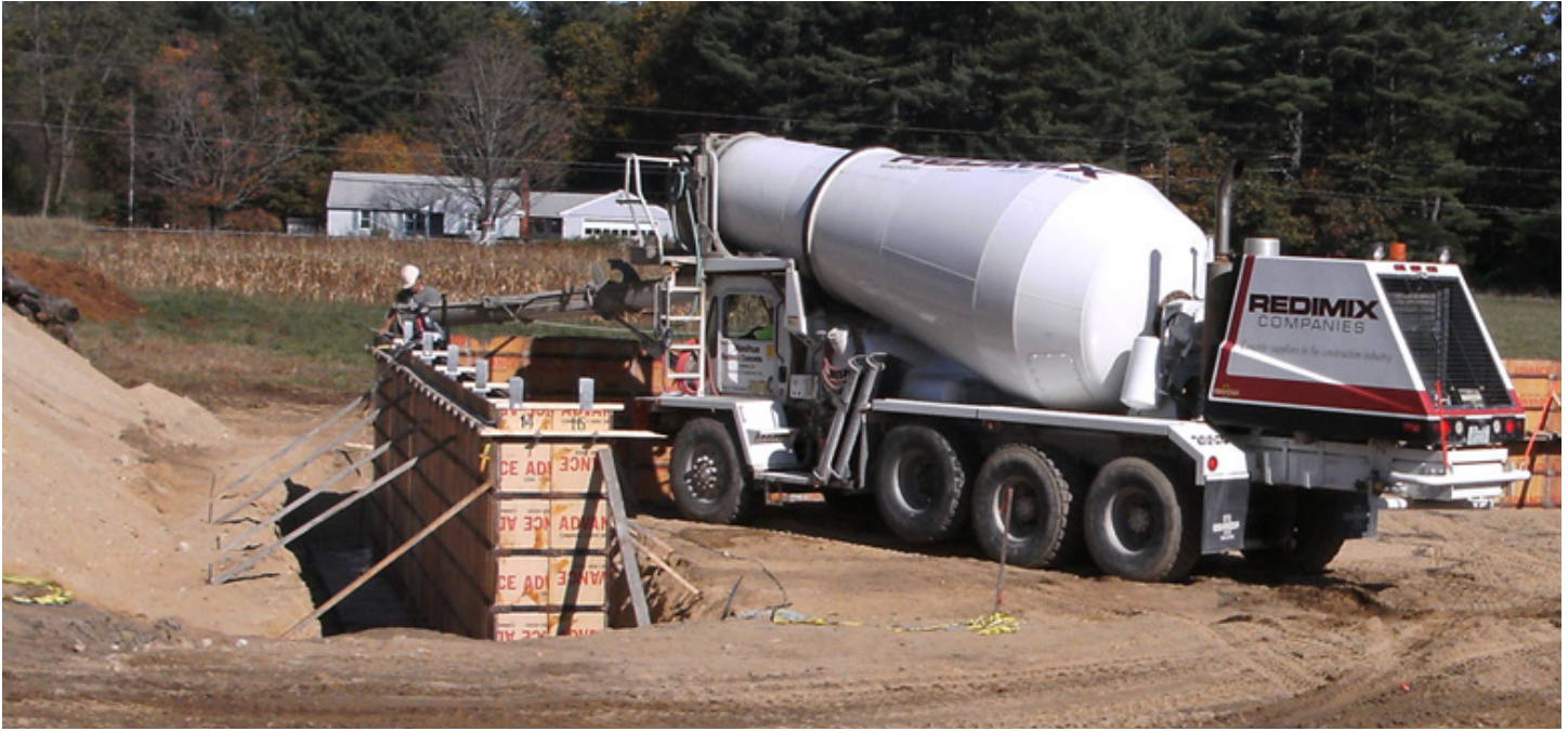
Figure 14: Sidewalls and Footings being poured at UNH Facility
