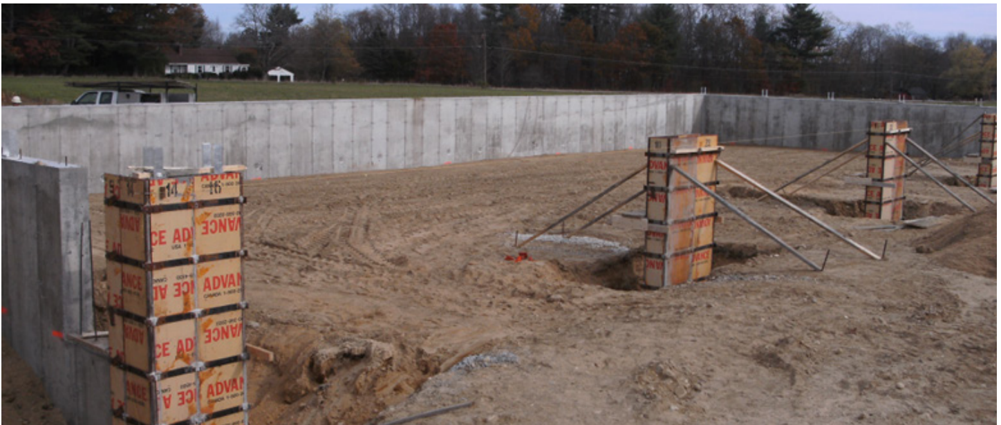
Figure 15: Concrete Piers at the UNH Compost Facility
