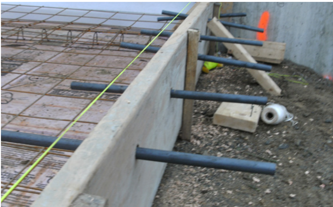
Figure 23: Concrete Slab-Connecting Dowels at UNH Composting Facility
