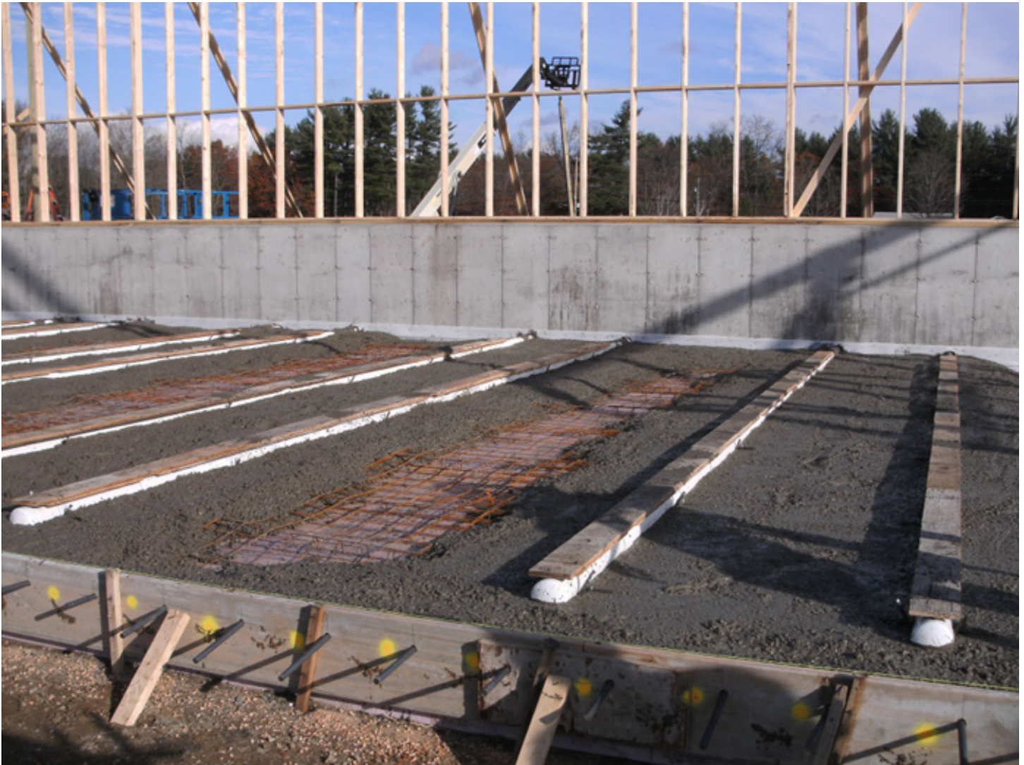
Figure 31: Concrete Pour for Main Composting Floor at UNH Facility
