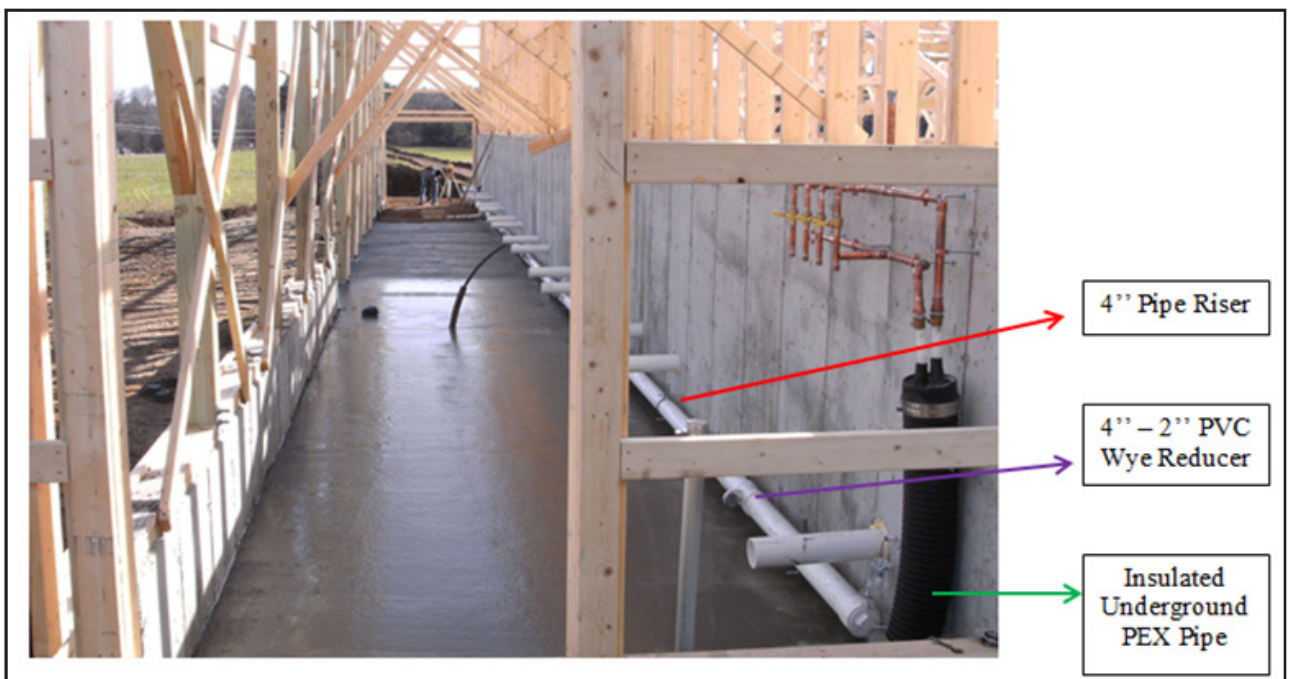
Figure 41: Specifications When Pouring Back Mechanical Floor
