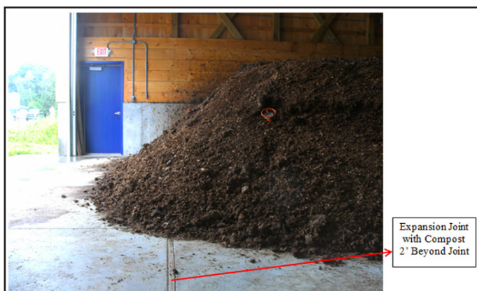
Figure 24: Expansion Joint between Primary Compost Floor and External Concrete Apron
