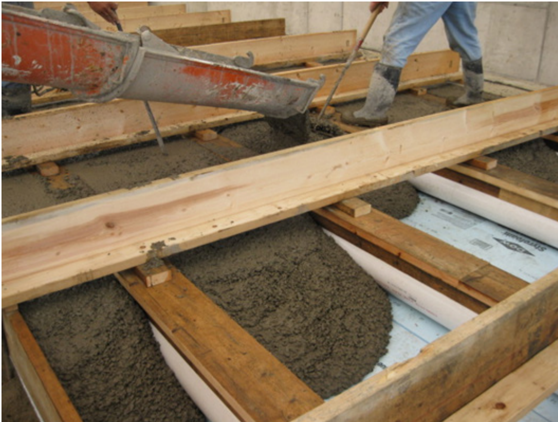
Figure 29: Alternate Cover Plate Form Setup (Jerose 2013)
