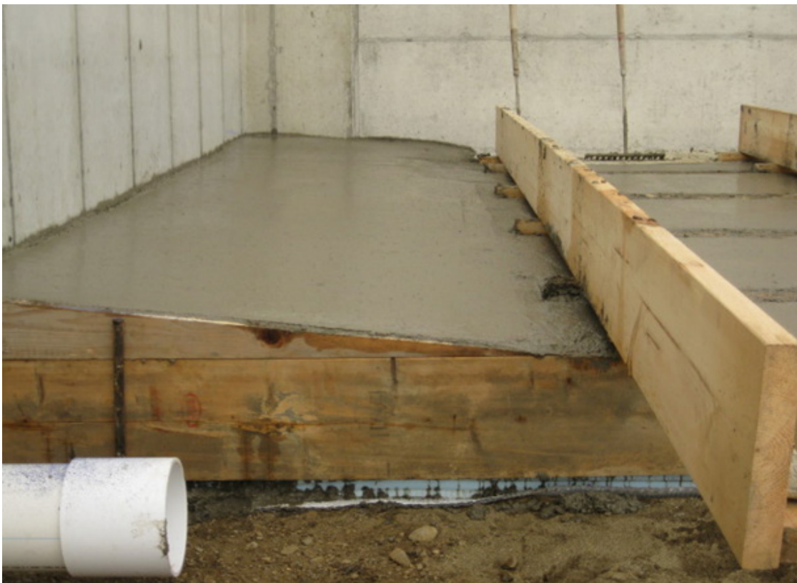
Figure 30: Alternate Cover Plate Form Setup (Jerose 2013)
