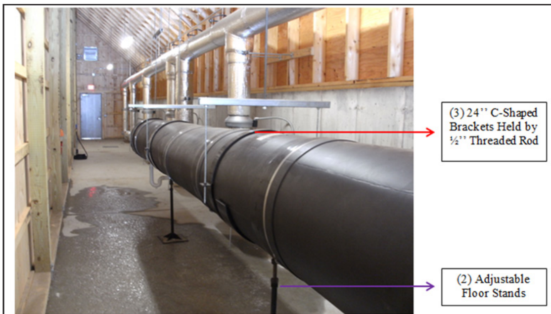
Figure 49: Support Structures for the Heat Exchange Unit
